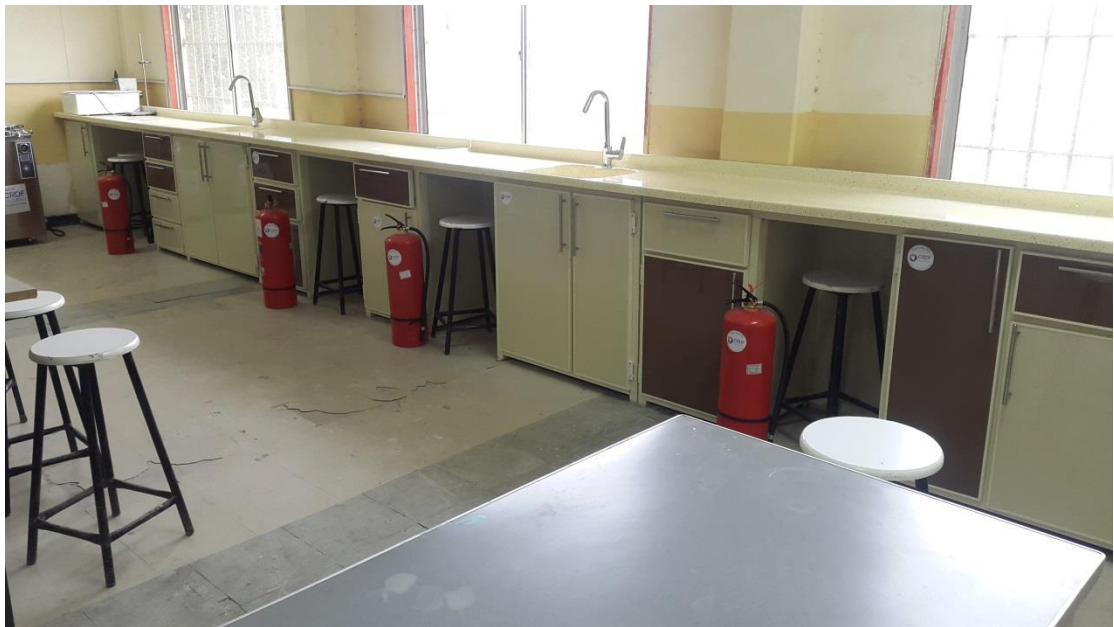
Working benches before and after installation
